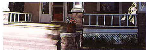
Inappropriate design – balusters too far apart.
