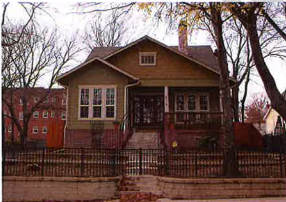
C.1.1 / C.1.2 While not a duplicate of existing houses, this house draws upon common characteristics of the district – raised crawl space, porch design, multiple front gables, siding patterns and grouped windows.
