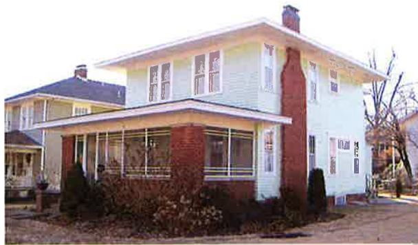
B.5.2 Example of enclosing a front porch with screens that maintain the character of the Prairie-Style house and can be removed in the future without damaging the historic brick columns.
