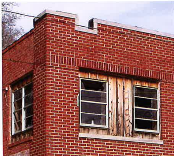
A.4.5 Inappropriate resizing of window openings
