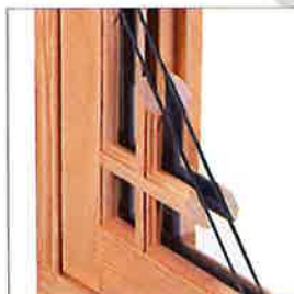
A.4.5 Exterior muntins (left), called “simulated divided light” or SDL, create a profile that more closely resembles historic windows than grids between the panes of glass (right). True divided light windows are also available and encouraged.
