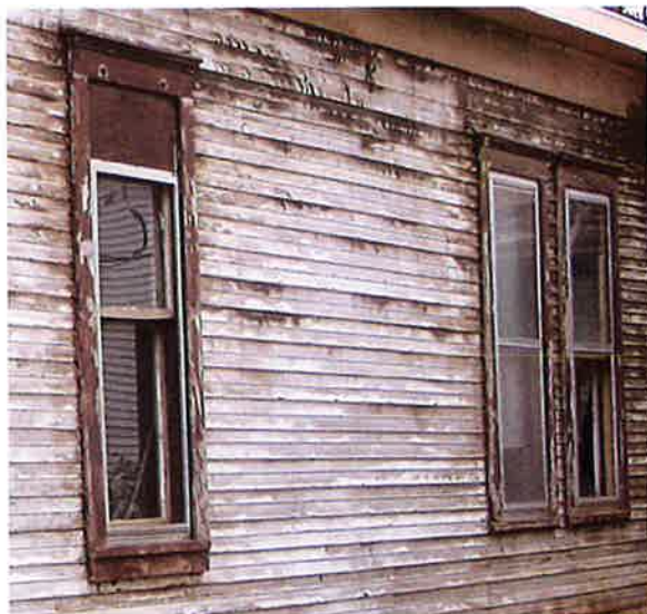
A.4.5 Inappropriate resizing (left window)
